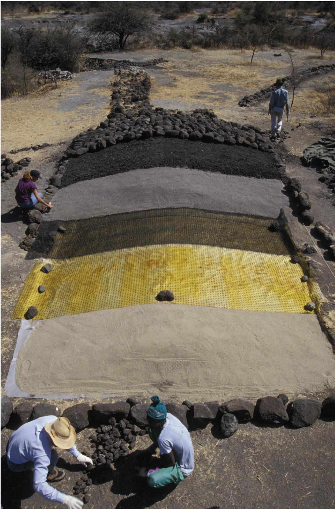
Figure 13 - After conservation, the Laetoli trackway was reburied under multiple layers of sand and geosynthetic materials, here showing several layers on the southern portion of trackway.
